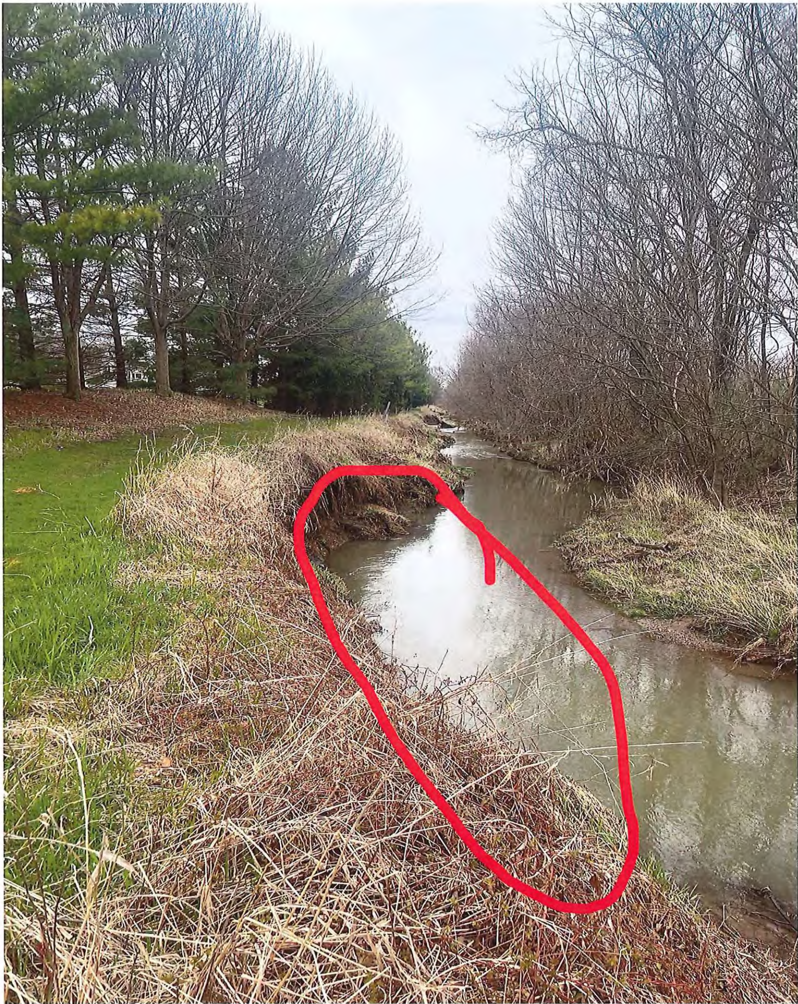
SITE E Project #25-006 Horn Ditch Brushing and Maintenance Project: erosion SITE E
