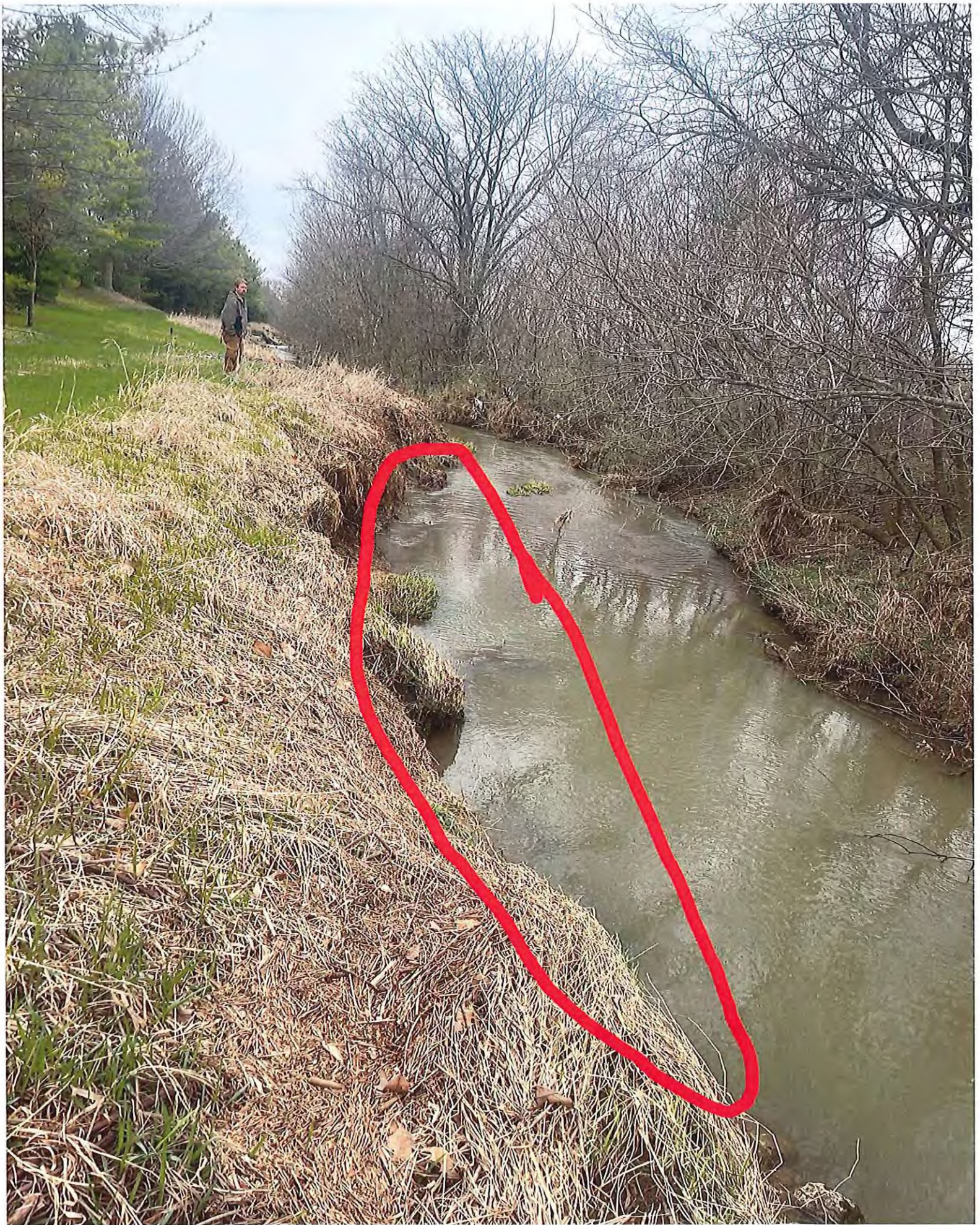
SITE D Project #25-006 Horn Ditch Brushing and Maintenance Project: erosion SITE D
