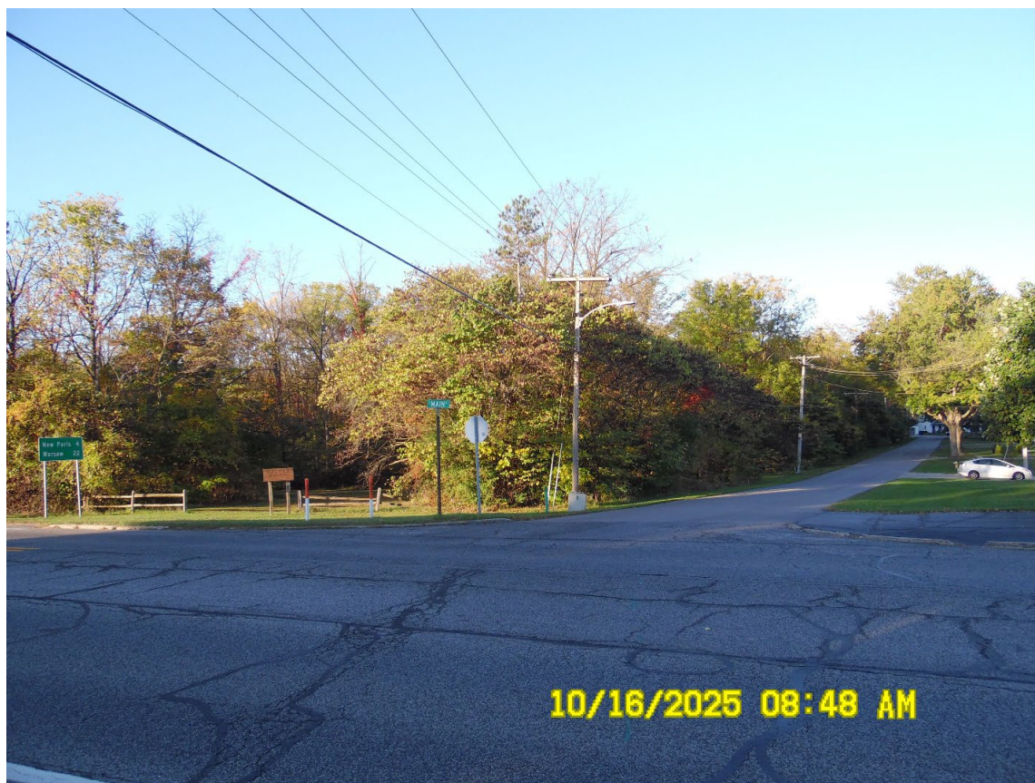
Looking southwest across Main Street at the northeast corner of the property
