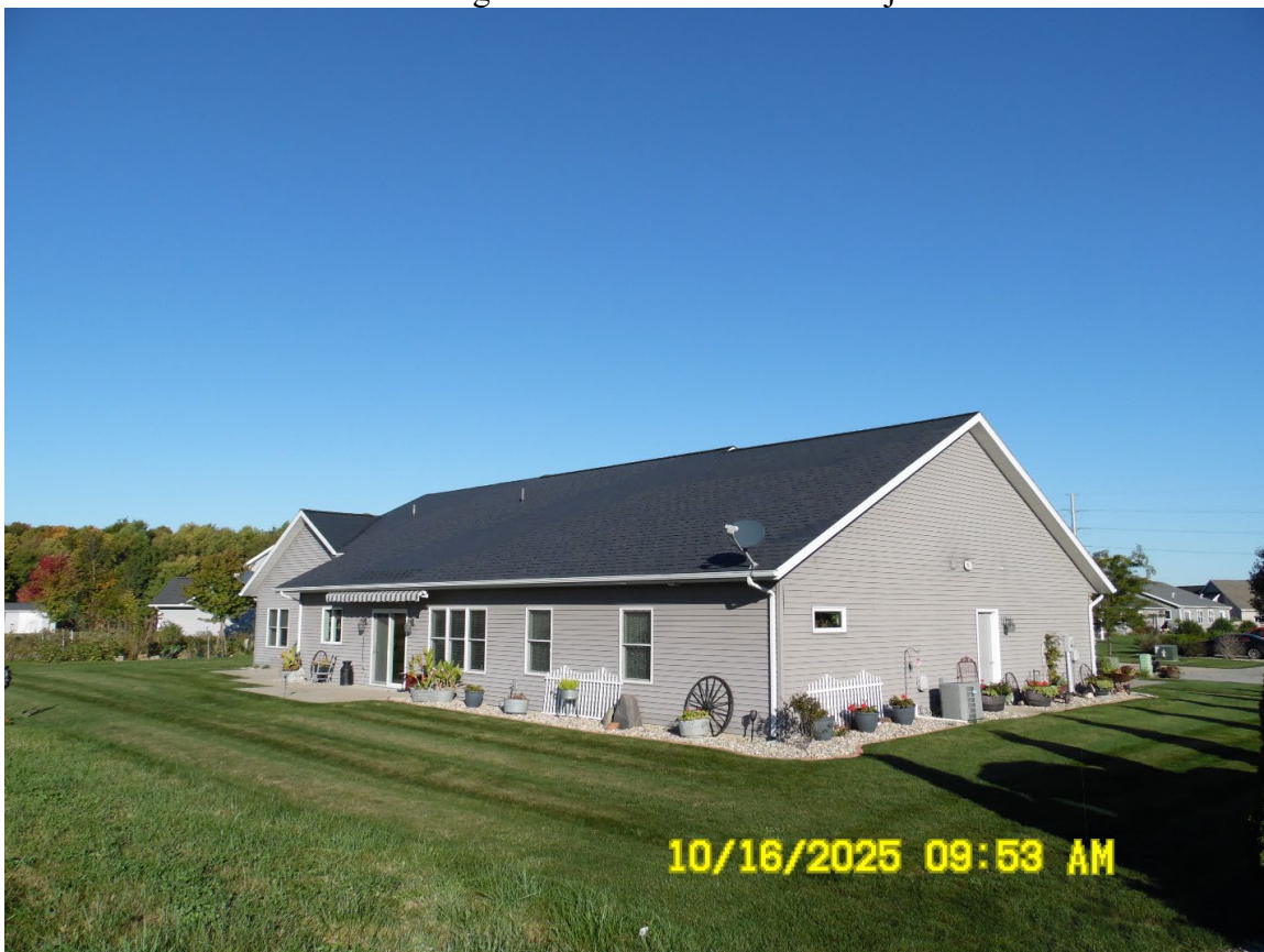
Looking northwest across rear of property
