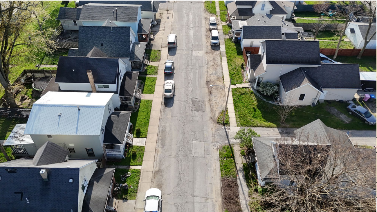
Oakridge Ave. looking East. Corridor is slated for full right-of-way Reconstruction including galvanized water service replacements, Storm Sewer, Sanitary Sewer, Streets, Curb & Gutter, and Sidewalk.
