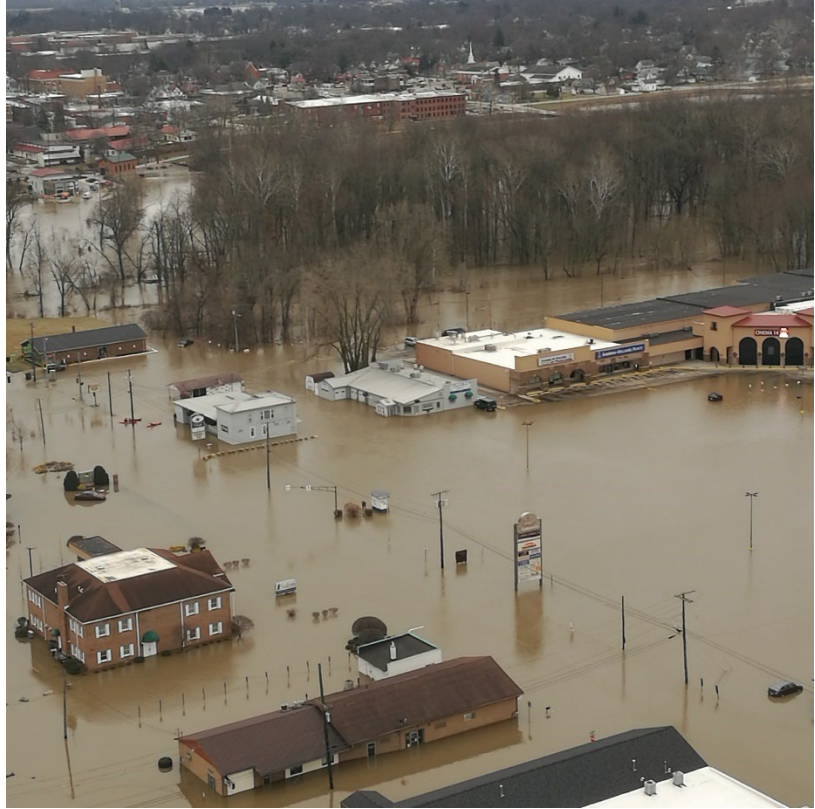
Figure 3-2: Flooding on Lincoln Avenue and Linway Plaza
