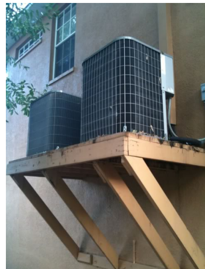
Figure 6-9: Example of Compliance with Flood Ordinance Requirements
