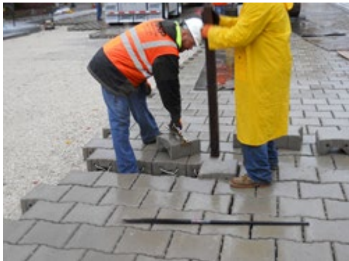
Figure 5-1: Installation of Permeable Paver System in Goshen
