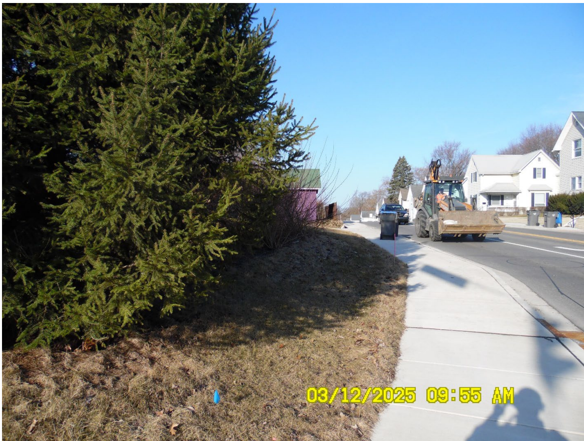
Looking west at location of proposed fence re-installation
