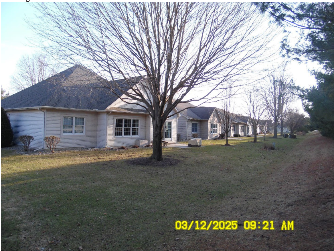
Looking northeast at rear of home
