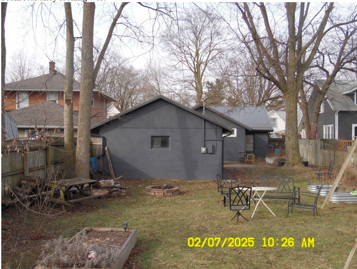
Looking west at detached garage
