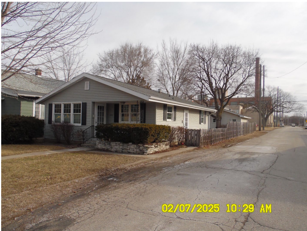
Looking east-northeast along New York Street
