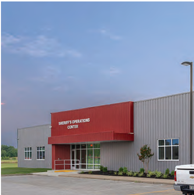
Vanderburgh County Sheriff's Operation Center
