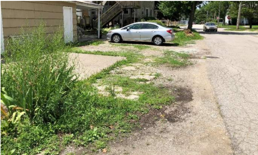
SW Franklin Street
