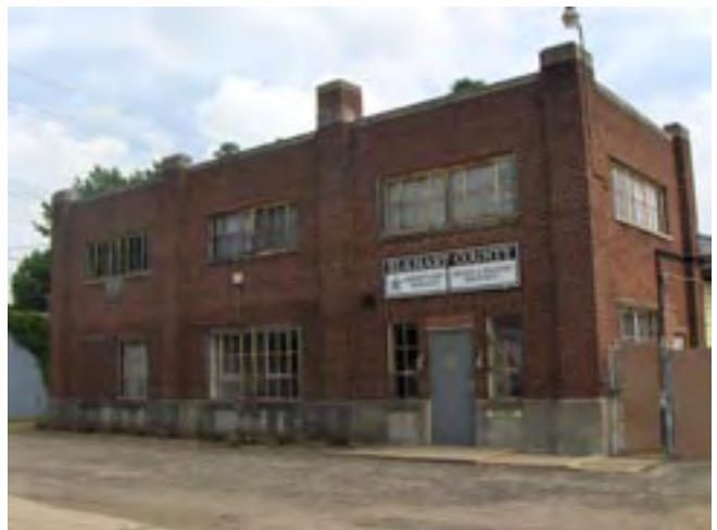
Elkhart County "Weights and Measures" Building
