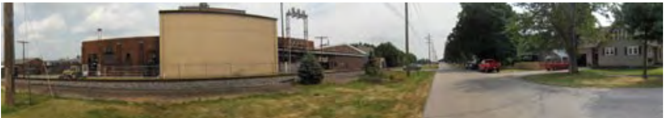
Panaramic views of 9th Street corridor
