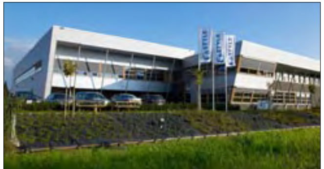
SMALL TO MEDIUM SCALE PRODUCTION FACILITIES
