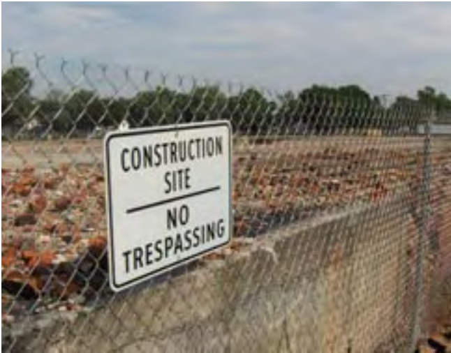
View of primary Western Rubber Site 1 under demolition
