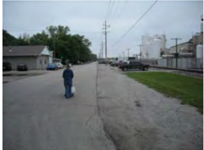
View of 9th Street, looking north near the Dairy Farmers of America (on the right). 9th Street lacks basic infrastructure components such as sidewalks, curb & gutter and stormwater drainage.
