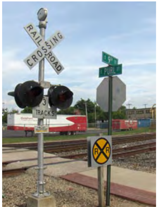
Intersection of 9th and Purl showing sidewalk improvements crossing the rail tracks.
