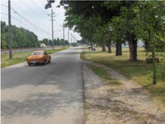
View of 9th Street looking south, near the intersection at College Avenue.
