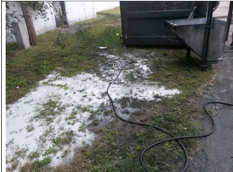
Observed white material being washed into City of Goshen Stormwater Inlet 507-3171
