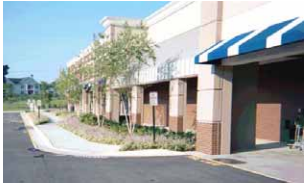
Example of Foundation Landscaping
