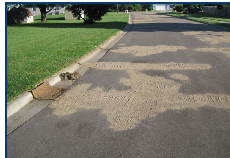
The Street Department uses inlet protection matting when they chip seal.
