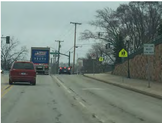
Figure 12. Existing bike lanes terminate unexpectedly in Elkhart. The bicycle lane in this photo terminated just west of this location.
