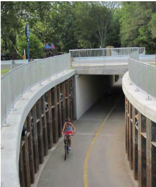
Figure 4. The 14-mile Mill Race Canal Area in Goshen includes the Shanklin Millrace Tunnel
