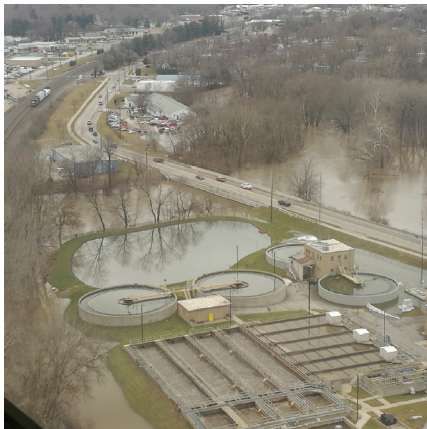
Figure 30: Flooding at the Wastewater Treatment Plant on February 21, 2018. The Elkhart River came within a few inches of overtopping the solid-waste holding lagoon (center of photo) and flooding wrapped around the south side (left of photo) of the property.
