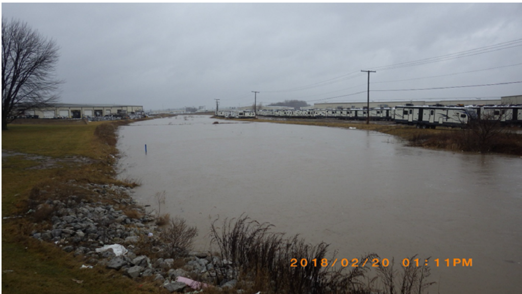
Figure 34: An image of the same area shown in Figure 33 during the 2018 February Flood illustrating how the floodwaters were contained within the two-stage ditch.
