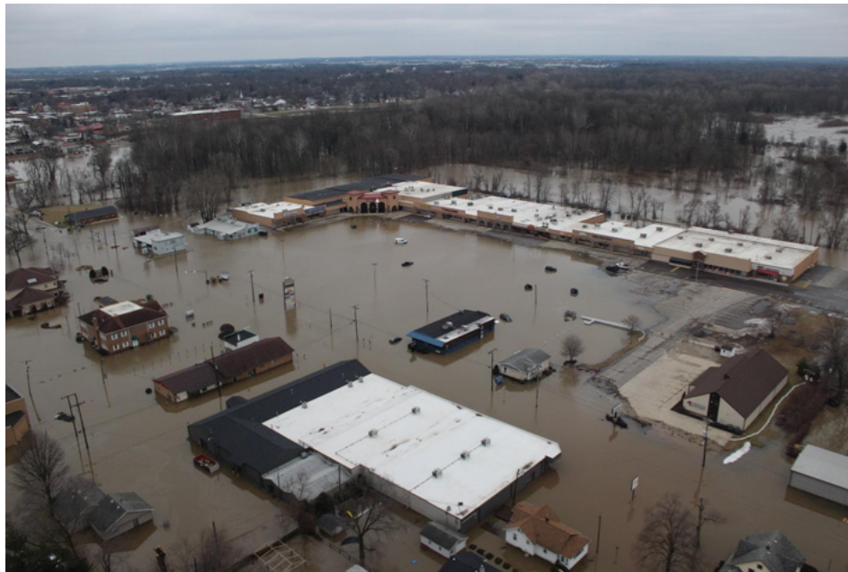
Figure 1: February 2018 floodwaters impacted businesses in Linway Plaza and along Lincoln Avenue.
