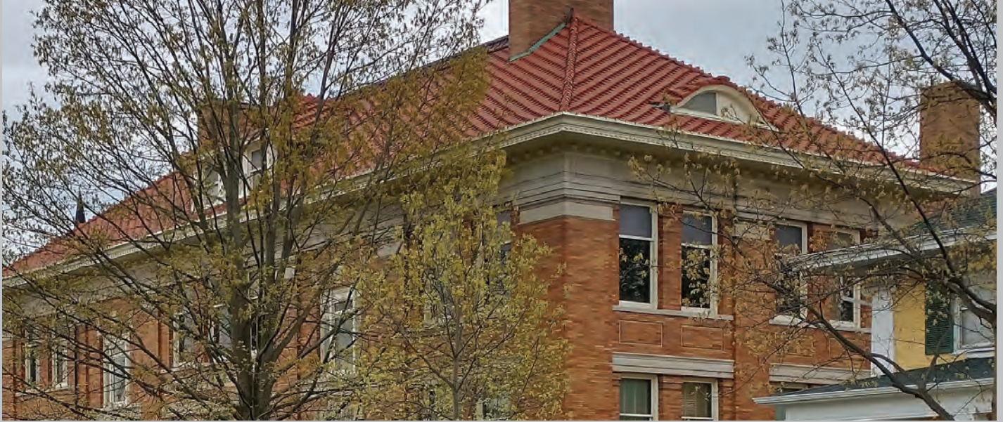
CITY ANNEX BUILDING
