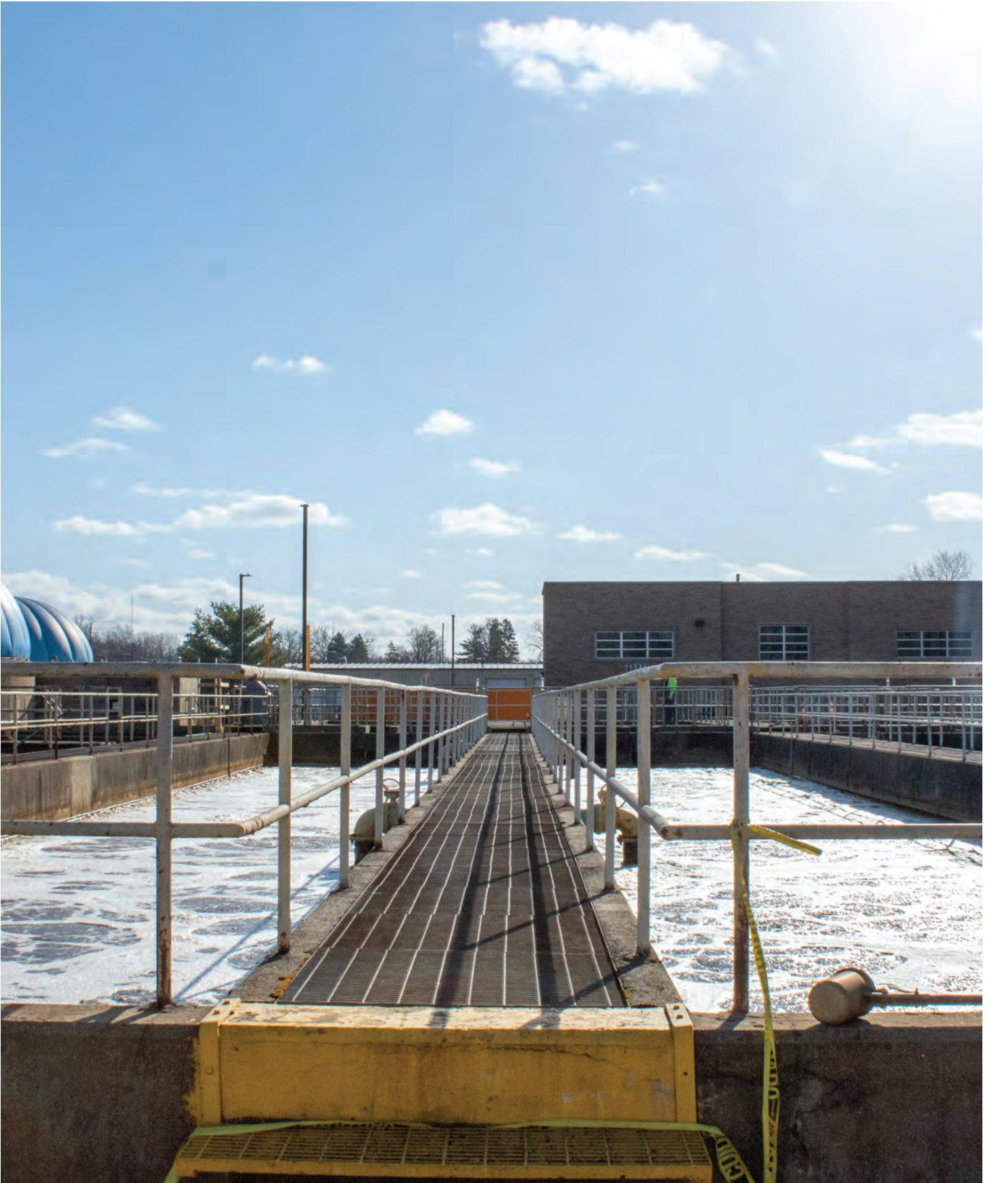
WASTEWATER TREATMENT PLANT
