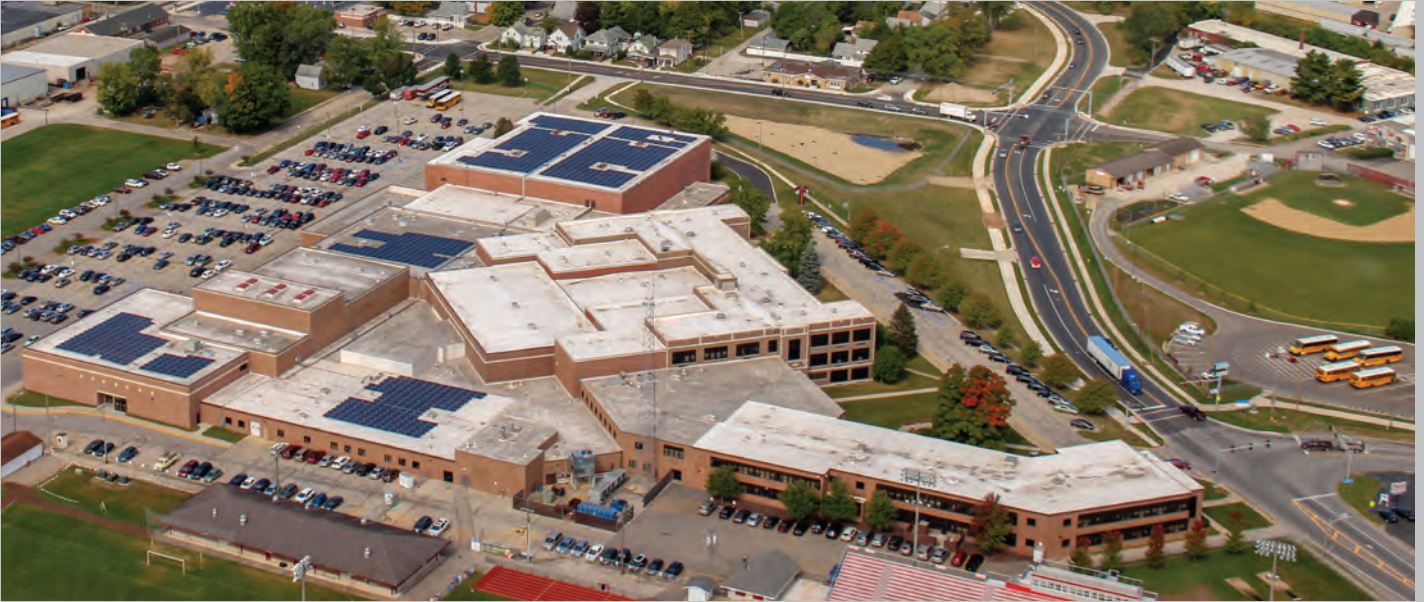
SOLAR PANELS AT GOSHEN HIGH SCHOOL
