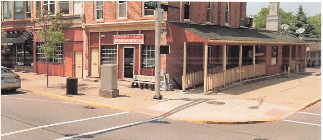
Figure 2 – Existing Exterior Ramp and Porch
