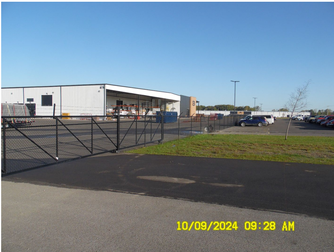
Looking northwest at shared fence crossing Lot 6 & 7
