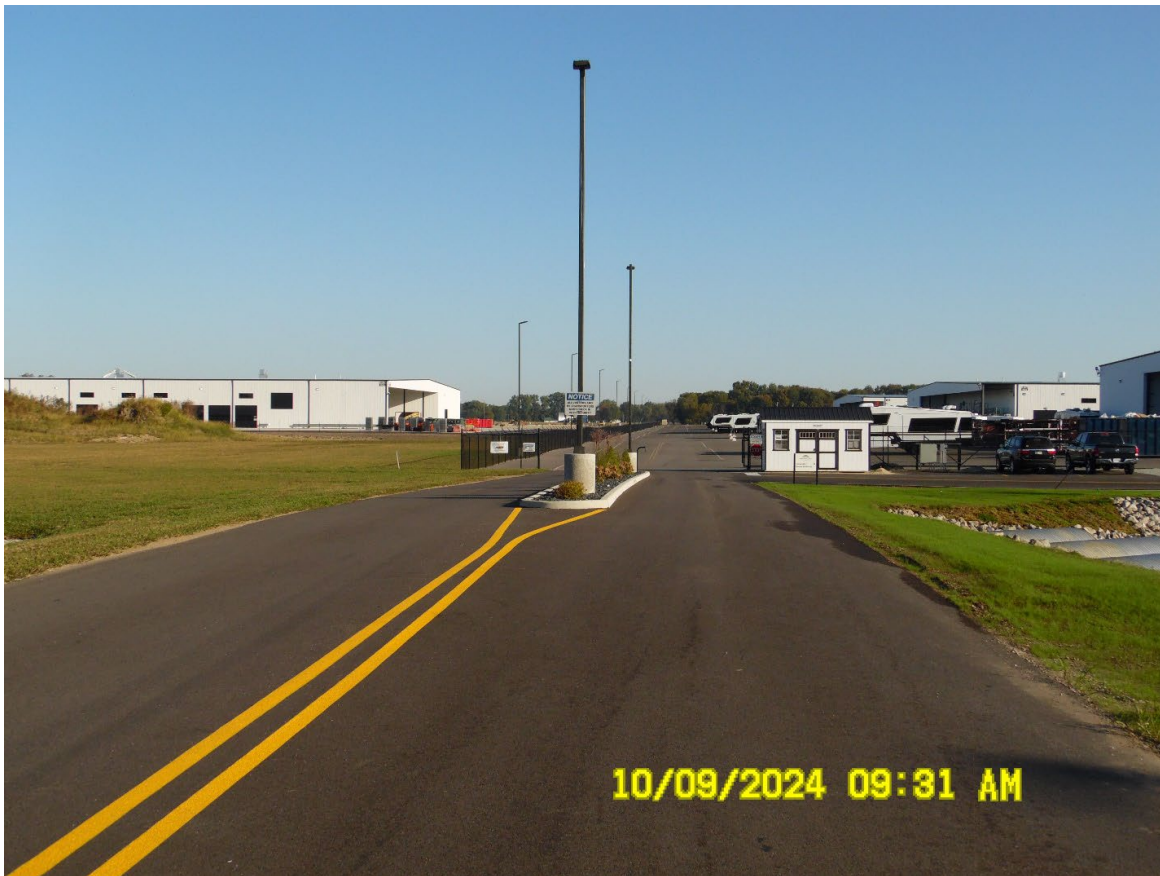
Looking north at shared access drive connecting all eight proposed lots
