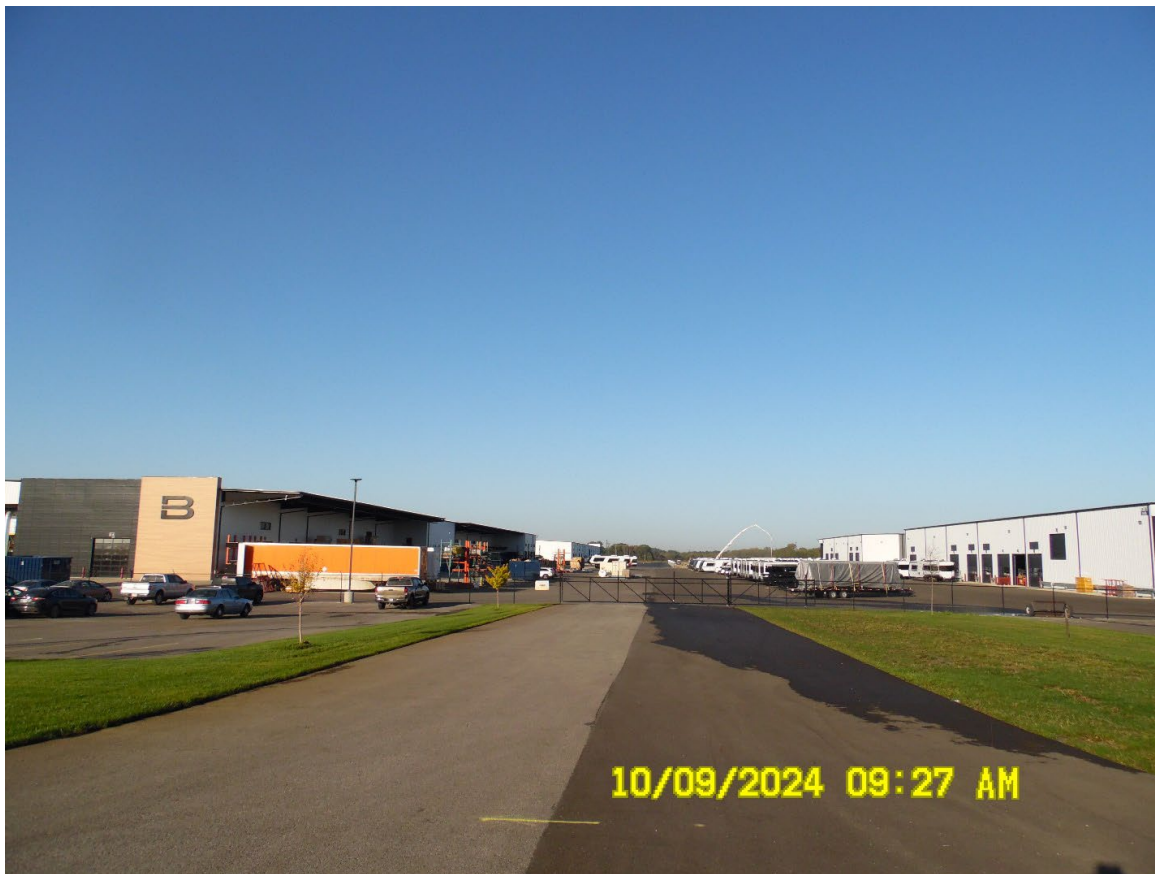
Looking west at the shared drive and 0' side setbacks between the proposed Lots 6 & 7
