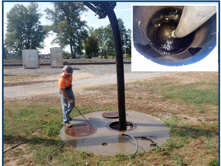
Quinn Grass of the Water & Sewer Department removes a lid from a STU. (Inset: Looking down into a structure as the Vactor truck runs.)
