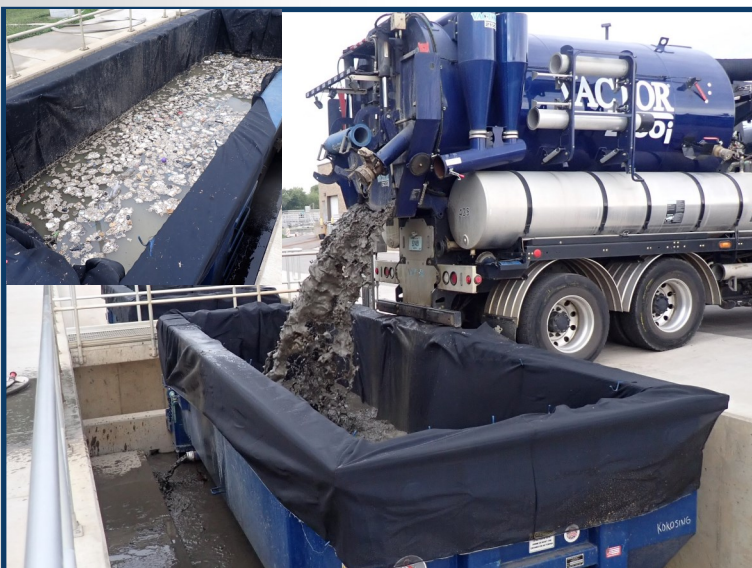
Materials captured by the STUs are dumped at the Wastewater Treatment Plant. (Inset: Debris left after a Vactor truck has emptied.)
