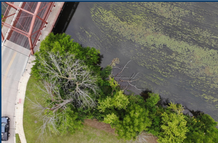
The Elkhart River at the Indiana Avenue Bridge
