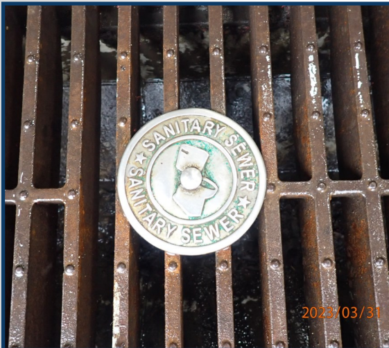
Drain marker used to denote where the water flows.
