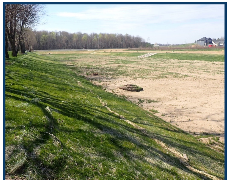
Basin #2, showing 1200 gallon drywells for more water storage.
