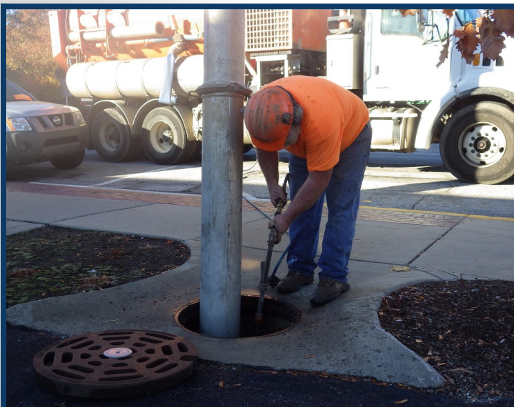
City of Goshen Sewer Department cleaning out a storm drain with a vactor truck.
