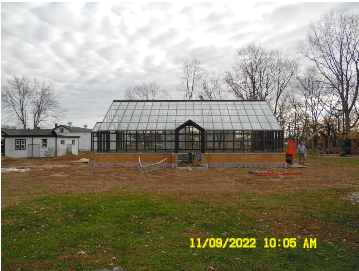
Looking east at greenhouse under construction approved in 2021
