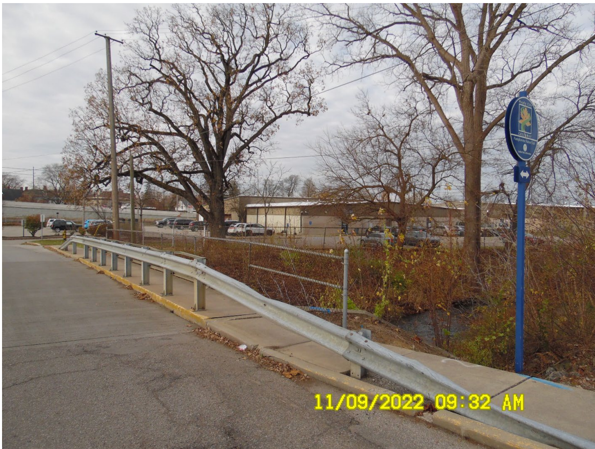
From intersection of Cottage and Bridge Street looking southwest across Rock Run Creek
