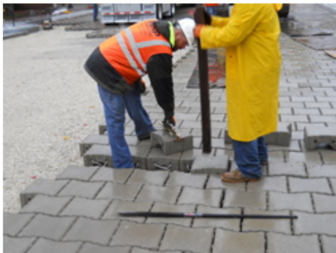
Figure 5-1: Installation of Permeable Paver System in Goshen
