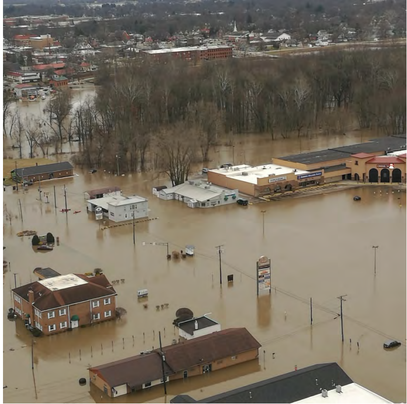
Figure 3-2: Flooding on Lincoln Avenue and Linway Plaza
