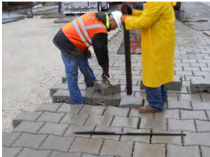
Figure 5-1: Installation of Permeable Paver System in Goshen
