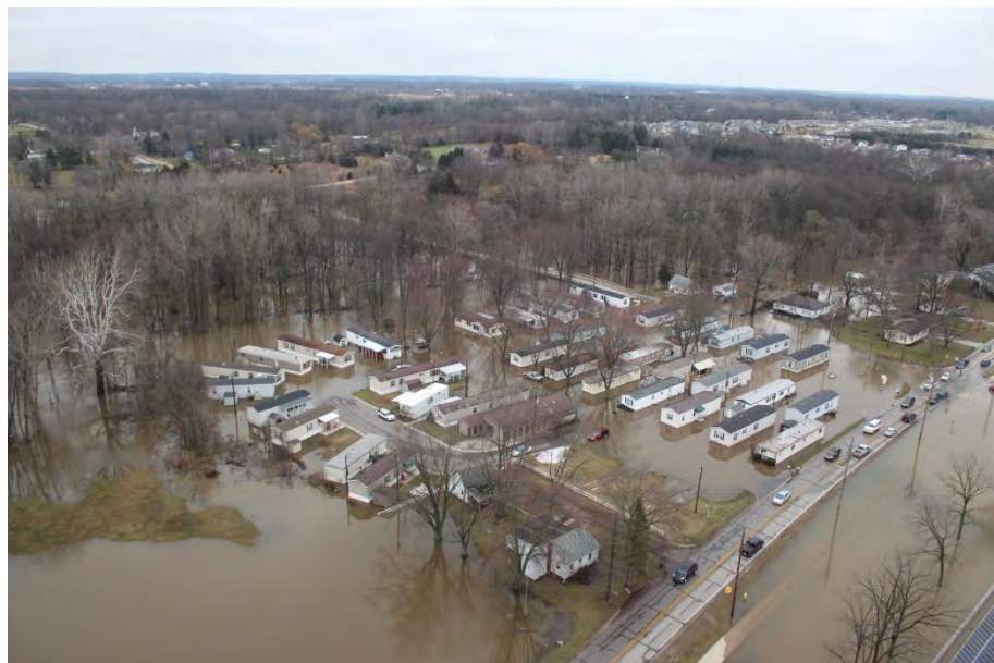
Figure 3-3: Flooding at Creekside Estates Mobile Home Park
