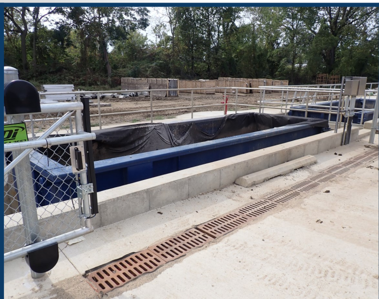
The dump station uses large, lined dumpsters to slowly drain water from the debris.
