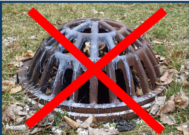
Hardened grease on a storm drain shows evidence of where dumping occurred.
