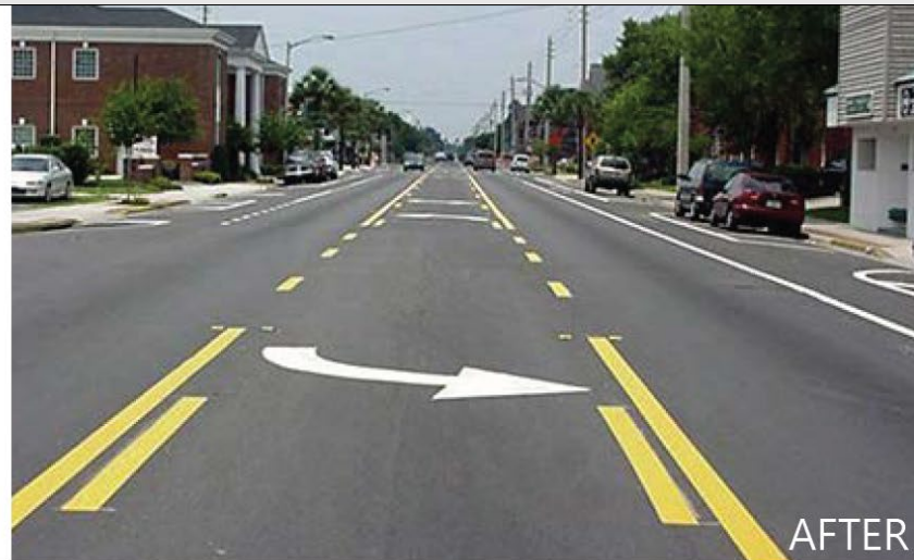
Before and after photos of a Road Diet project.
