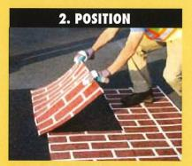
Position the TrafficPatterns™ material according to layout provided.
