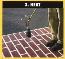
Heat TrafficPatterns™ with a propane heat torch then chisel test to verify proper bond.
