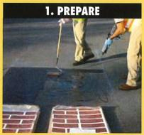
Remove debris. Ensure no moisture is present and apply TrafficPatterns™ Sealer according to instructions provided.
