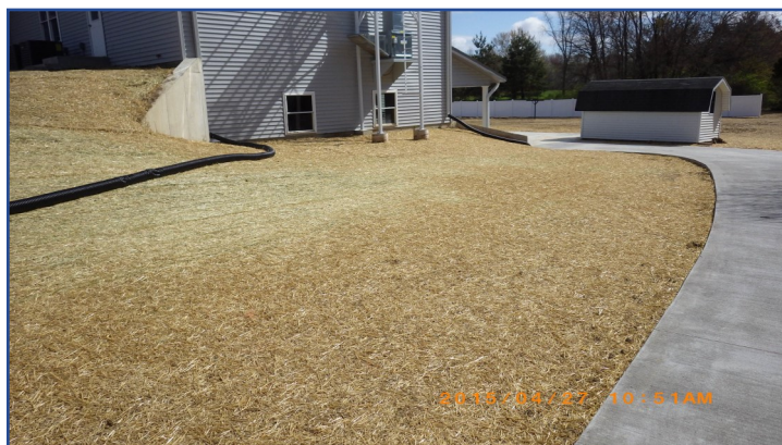
All bare soil has been covered with a temporary mulch because it reduces the chance for erosion to happen.
