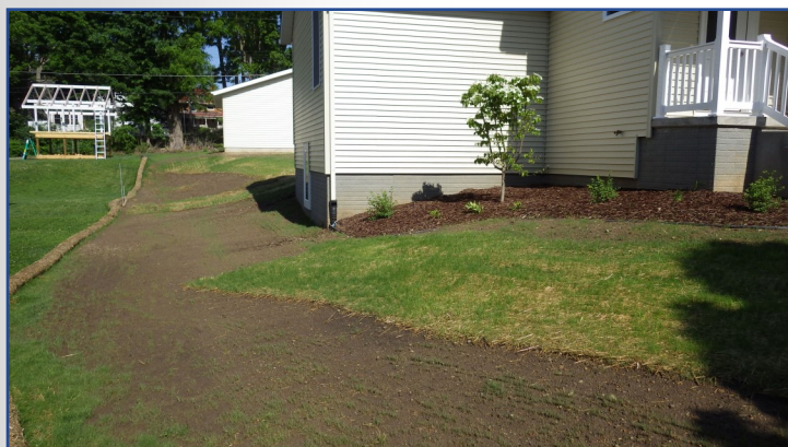
Notice how vegetation is growing better where the straw erosion control blankets were used.
