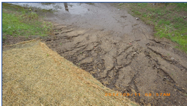
Erosion of the bare soil is clearly visible where the straw erosion control blankets ended.
