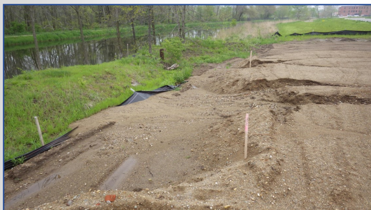
The bare soil eroded and overtopped the silt fence while the existing vegetation stopped the sediment before it reached the water.
