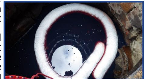
An absorbent boom is being used to absorb diesel fuel that flowed into a storm drain.
