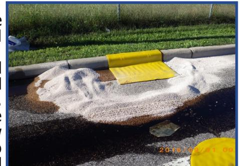
Two measures were used to stop diesel fuel from entering a storm drain after an accident.
