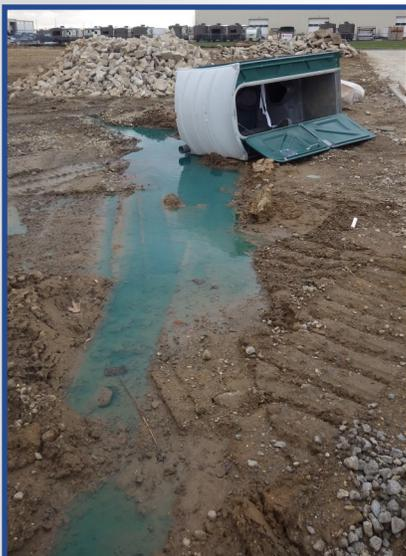
Chemicals and contaminated soils from this tipped over portable toilet will need to be removed and disposed of properly.
