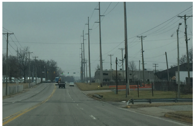
Figure 11. Some roadways in low-density areas in Elkhart lack sidewalks and marked crossings.
