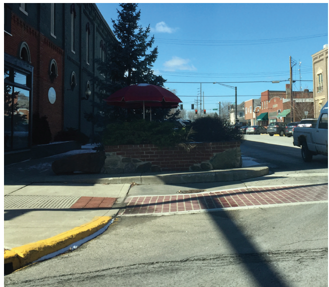
Figure 6. A decorative crosswalk and curb bumpout in Goshen.
