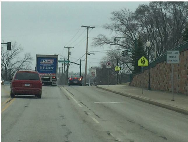
Figure 12. Existing bike lanes terminate unexpectedly in Elkhart. The bicycle lane in this photo terminated just west of this location.
