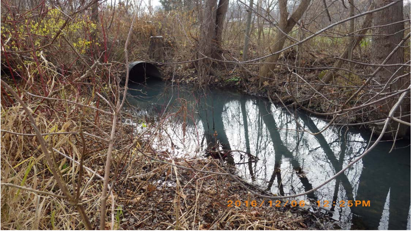
Discolored water in Wellington Ditch extended north of Waverly Avenue. The extent of the discolored water was not explored beyond this point. (The culvert in the picture goes under Waverly Avenue.)
