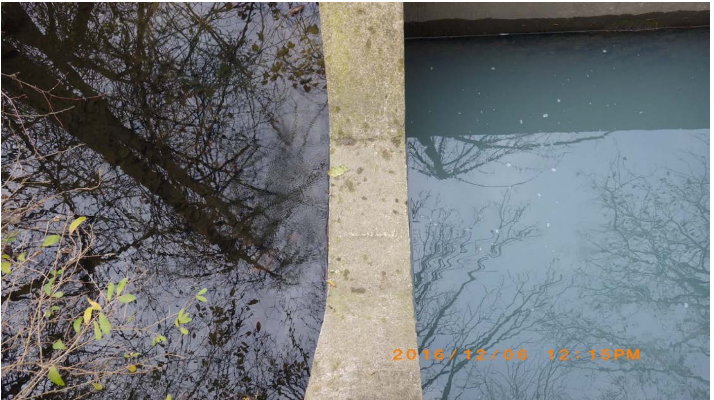
Here is a comparison between the water coming out of the College Avenue outfall and just upstream of the concrete structure.
