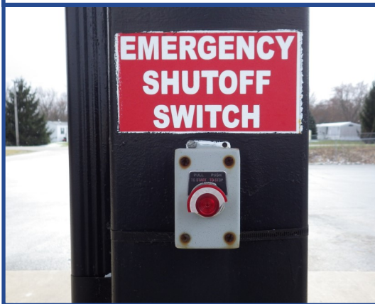
Emergency Stop Button—Located near each fuel pump.
