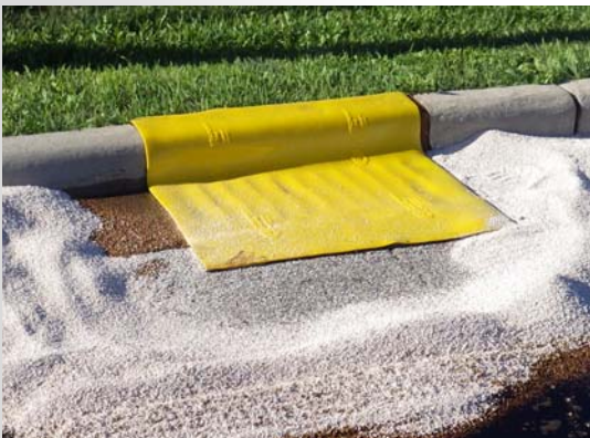
Left - A Drain Blocker Mat and oil-dri berm keep diesel fuel from flowing into a storm drain. Right - Sunpro employees work to clean up spilled diesel fuel from the roadway.
