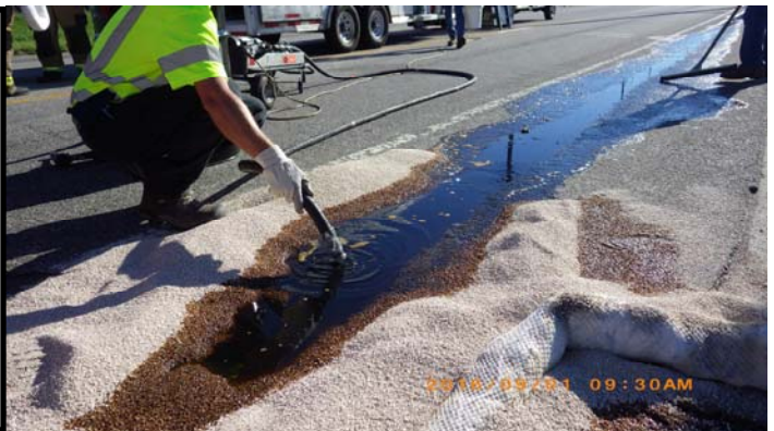
Left - A Drain Blocker Mat and oil-dri berm keep diesel fuel from flowing into a storm drain. Right - Sunpro employees work to clean up spilled diesel fuel from the roadway.
