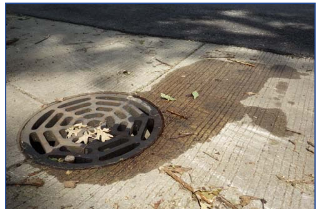
An abandoned vehicle with an engine leak was parked next to a storm drain inlet.
