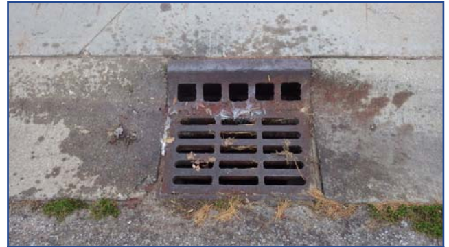
A resident dumped used oil/grease in and around a storm structure.
