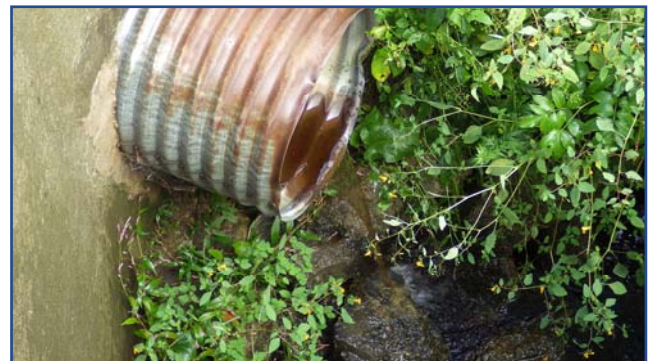
Tea colored water coming from an storm sewer outfall pipe.
