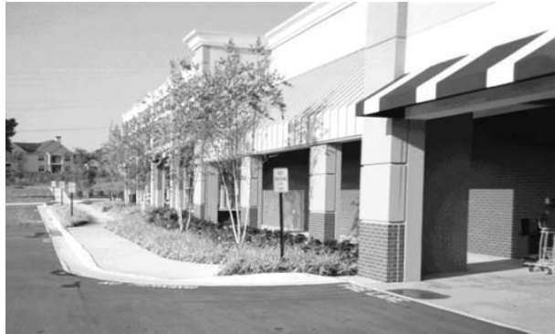
Example of Foundation Landscaping
